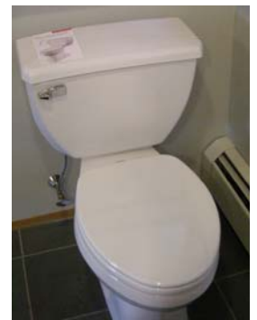
The HET at Riverbend uses only 1.1 or 1.6 gallons per flush, saving water, money, and energy!
