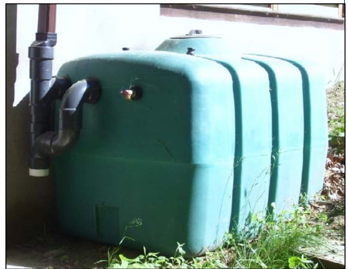
Rainwater Recovery, Inc. provided a 200-gallon cistern that collects rainwater from a downspout for use on the property.
