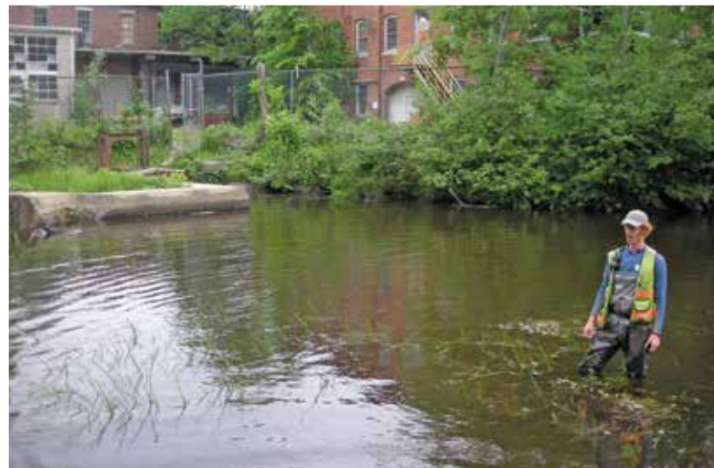
Nick Nelson (Inter-Fluve, Inc.) wades into the Ipswich River upstream of the South Middleton Dam to inspect the aging dam. The inspection is part of a detailed survey of the dam and the river necessary to develop the construction plans for the dam's removal in 2016.
