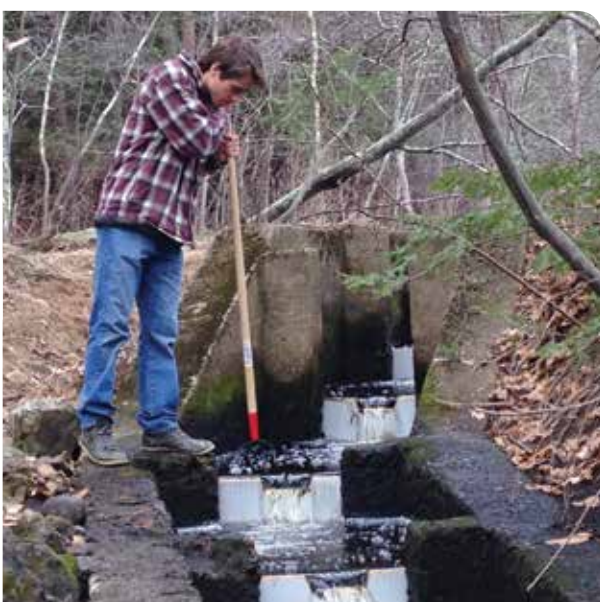
Alex Walsh, a Trout Unlimited volunteer, maintains the new board system at the Willowdale fish ladder which allows fish to more easily swim up the ladder. Photo: Chett Walsh
