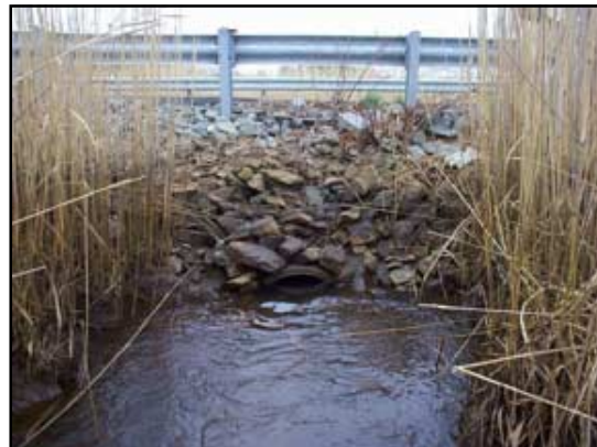
The top of the 20-inch pipe is barely visible here; although Phragmites lines the seaward channel near the roadway berm, salt marsh dominates the seaward area.
