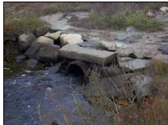
This 2-foot culvert opening passes flow under Fisk Street between Weir Creek and Kelleys Pond.
