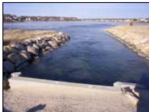
Rock armored upstream channel flowing into Little Pond.
