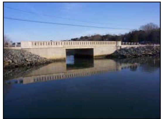
Seaward side of Millway Road bridge seen at high tide.
