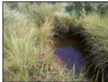
This pool of water submerged the 18-inch opening on the seaward side of Cranberry Lane.
