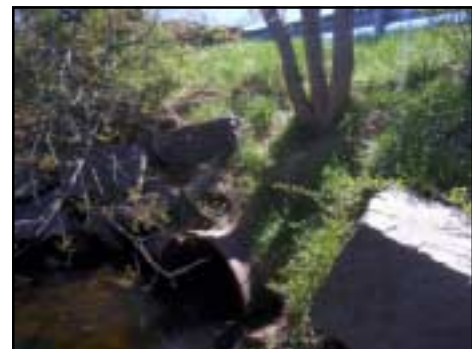
The 3-foot pipe opening is visible here upstream of Wilder Dike.
