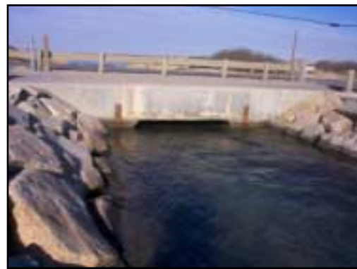
Seaward culvert opening nearly submerged by the rising high tide.
