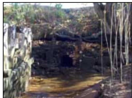
Phragmites , visible in the foreground, is the only thing growing in the exposed mud near this upstream pipe opening.
