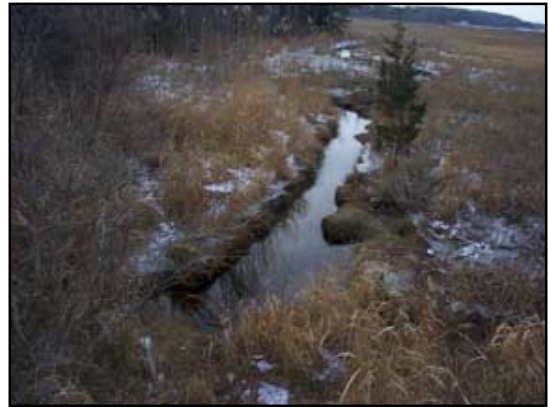
Phragmites and shrubs are taking hold in the salt marsh near the seaward opening of the pipe.
