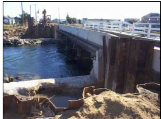
The Craigville Beach Road bridge undergoing reconstruction in the fall of 2000.
