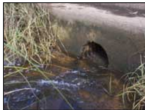
This 16-inch corrugated metal pipe set in the concrete headwall passes the flow of the Red River under Deep Hole Road.
