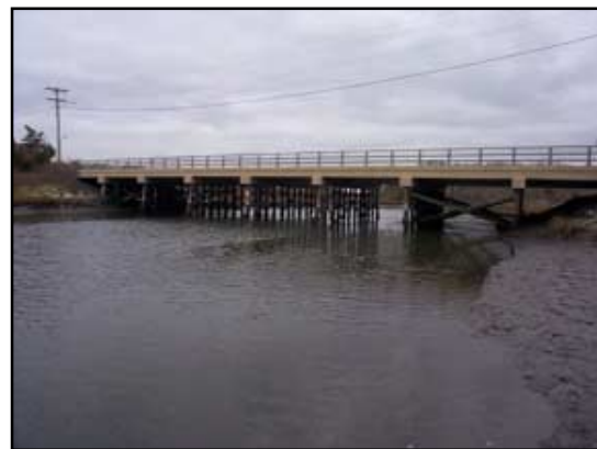
This 155-foot bridge span carries Route 28 across the Herring River.
