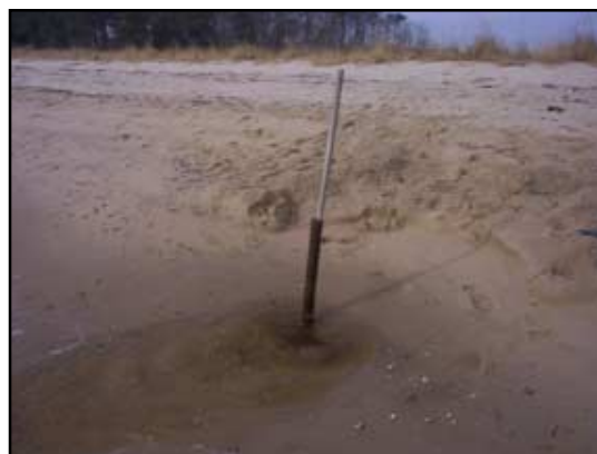
This stick marks the location of the seaward culvert opening.
