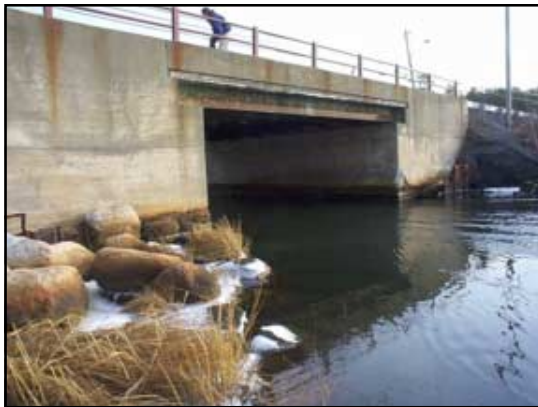
Seaward side of the concrete box opening under Meadow Neck Road.
