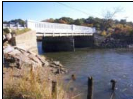
This 60-foot long stone bridge moves Route 6A traffic over Scorton Creek.
