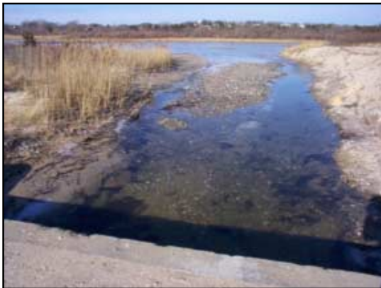
Upstream channel with fringe Phragmites and minor scour visible.
