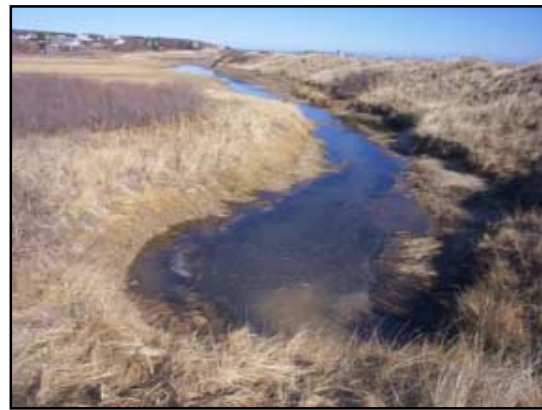
Even through the clear water the seaward pipe opening is not visible, however scouring is visible on the sides and bottom of the channel.
