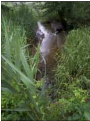
Phragmites and shrubs are visible in the upstream area as seen from the upstream side of the pipe.
