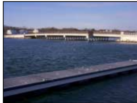
Seaward side of the bridge as seen from the Green Pond Town Landing.
