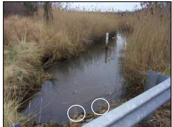
Two pipes are barely visible through the stagnant, murky waters by Kildee Road; Phragmites lines the seaward channel.
