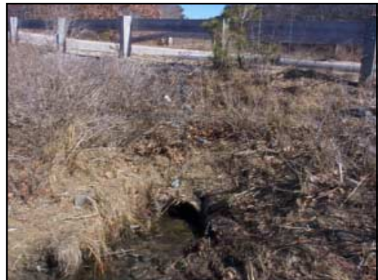
16-inch seaward pipe opening under Teaticket Path.
