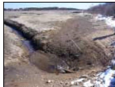
Scour, erosion, and vegetation die-off are severe in the seaward salt marsh adjacent to site BR-2.
