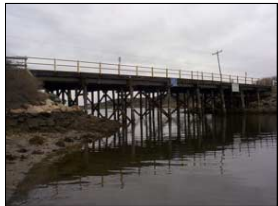
Lower County Road crosses the Herring River via this 90-foot bridge.
