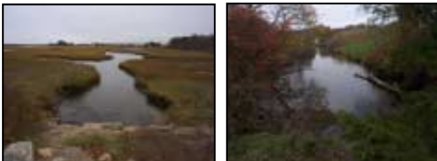
As evidenced by these two photographs, the vegetation changes significantly from the seaward (left) to upstream (right) sides of the Fisk Street tidal crossing.
