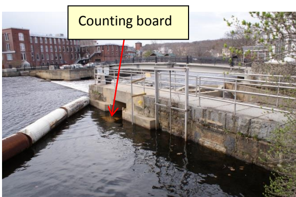
Figure 6. Counting location at the top of the fish ladder on the Ipswich Mills Dam. Note the location of the counting board in relation to the fish ladder visible in the background.
