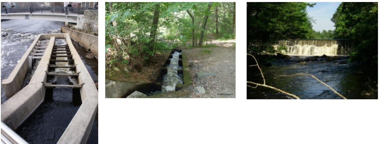
Figure 2. From left to right: Ipswich Mills Dam denil fish ladder, Willowdale Dam notched weir-pool fish ladder and Bostik dam with no fish passage.
