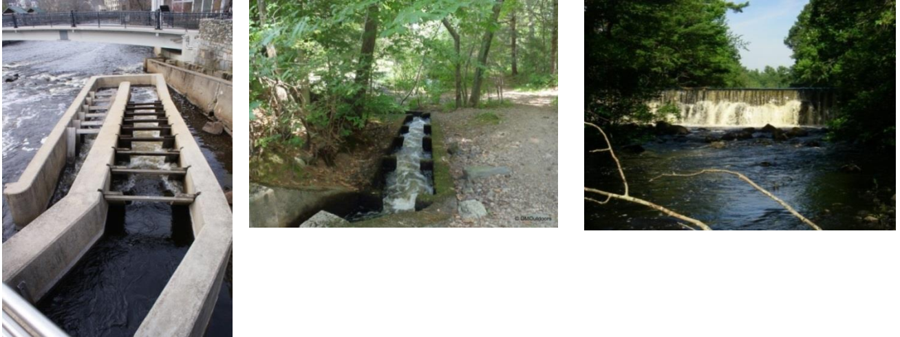
Figure 2. From left to right: Ipswich Mills Dam denil fish ladder, Willowdale Dam notched weir-pool fish ladder and Bostik dam with no fish passage.
